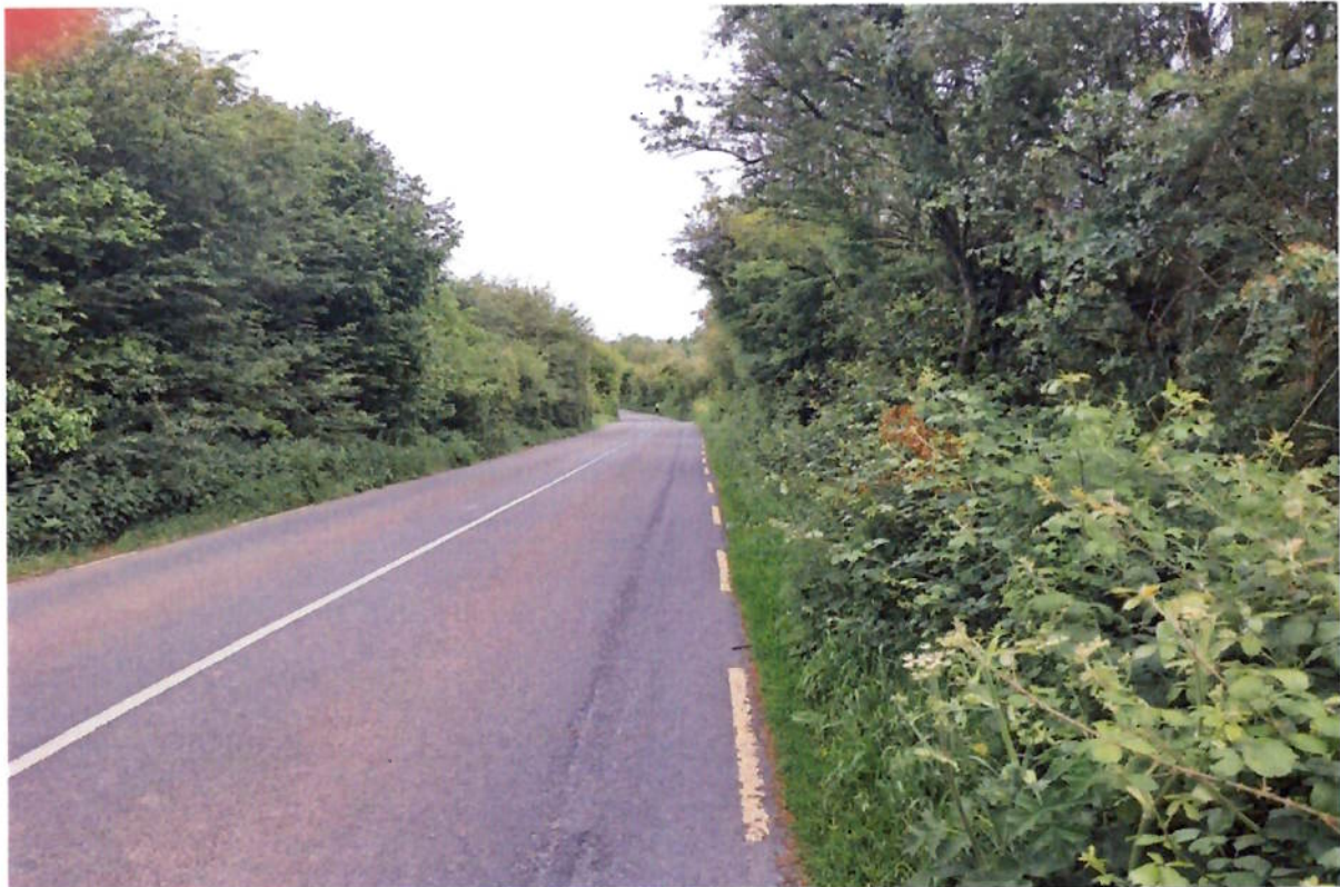
Image taken 117m on Sharavogue Railway Bridge from site entrance
